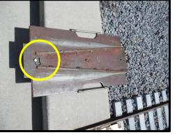
Hole is for pin that holds the transfer plate in place while moving equipment.
