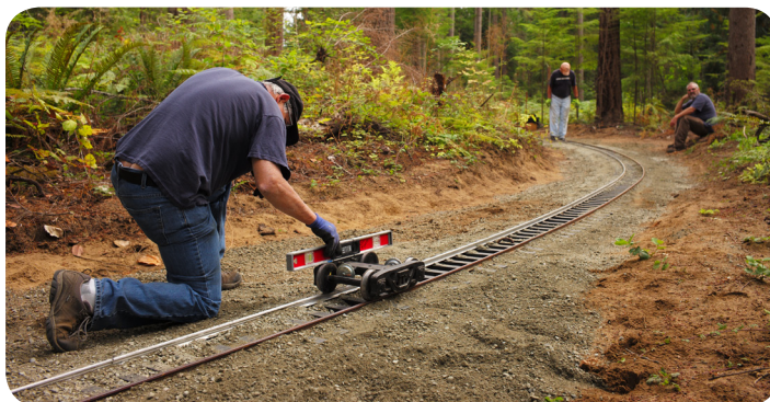
Don Rogers checking the slope on the new wye track
