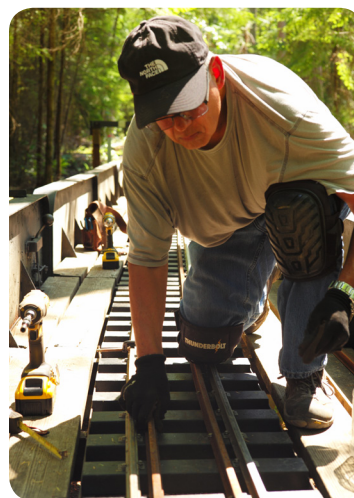
Don Rogers installing guard rails on the steel bridge
