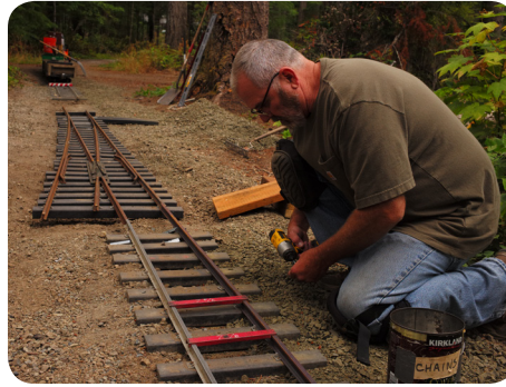
Tom Huffman working on the installation of the first switch for the wye
