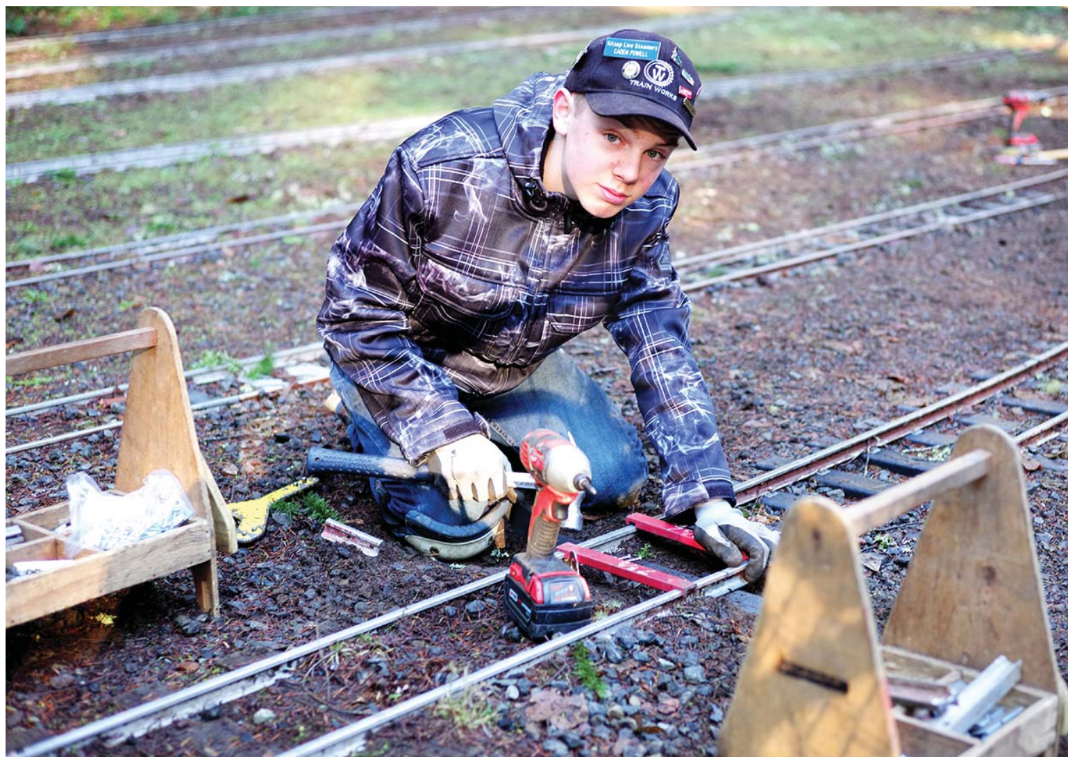
Caden Powell replacing old ties in the KLS Yard. Photo by Bill Hartung
