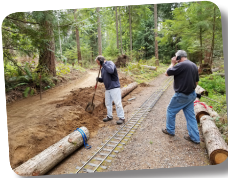
Building the log retaining wall for the Wye
